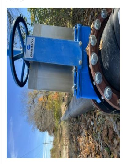
The most crucial piece of infrastructure for the canal is the pipe pictured above. This 16-inch line, powered by a 200-horsepower pump, supplies about three million gallons of water to the canal every day. The water is extremely clean and even wards off mosquitoes due to its composition! To open or close the valve, it takes about fifteen minutes of walking around and around the valve with a four-foot pipe wrench.
